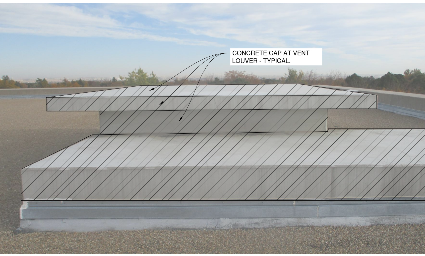
E COATED CONCRETE LOUVER VENT CAP & CURB - TYPICAL NOTE: SIMILAR - ACTUAL CONDITIONS MAY VARY (N.T.S.)
